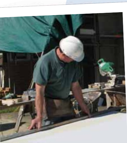
Below: Framework's participation with Habitat for Humanity
